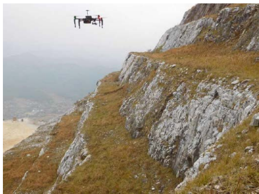
残壁の浮石点検
